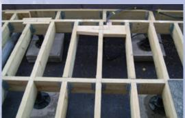
Contractors will lay the joist frame onto the flat heads at around 600mm centres. The timber can be spot bonded, fixed with a wood screw or simply be freestanding; so long as the edges are secured. By this method none of the timber is left in standing water, reducing any chance of rotting.
