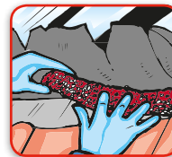
Repairing torn lead flashing
