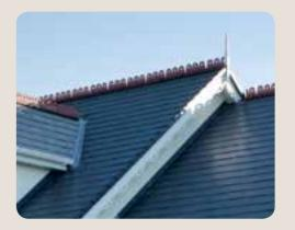
Our concrete Ornamental Ridges and Finials are compatible with mortar bedding, dry fix and ventilated systems, enabling a complete roof to be easily achieved without compromising good looks.
